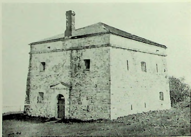
MAGAZINE BUILDING AT FORT NIAGARA, N. Y.
